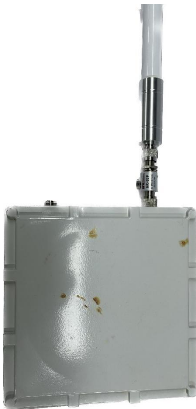
Figure 12 Install surge protector and LoRa antenna
