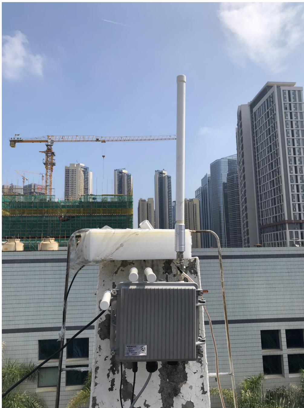
Figure 4-25 Wall mounting
